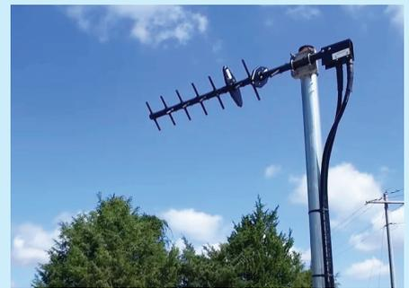
A technician mounts the conduit to a transformer and runs a LMR600 cable down and terminates it at the electrical box, where the modem is mounted, just beneath a communications card. Technicians simply plug in power, terminate two connections, then connect the Ethernet port—a simple, fast installation.
